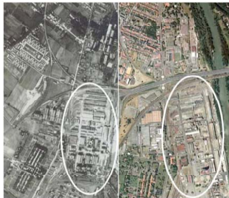
France, ONIA/AZF plant and neighborhoods in the 1930's and in 2001. Source: IGN
